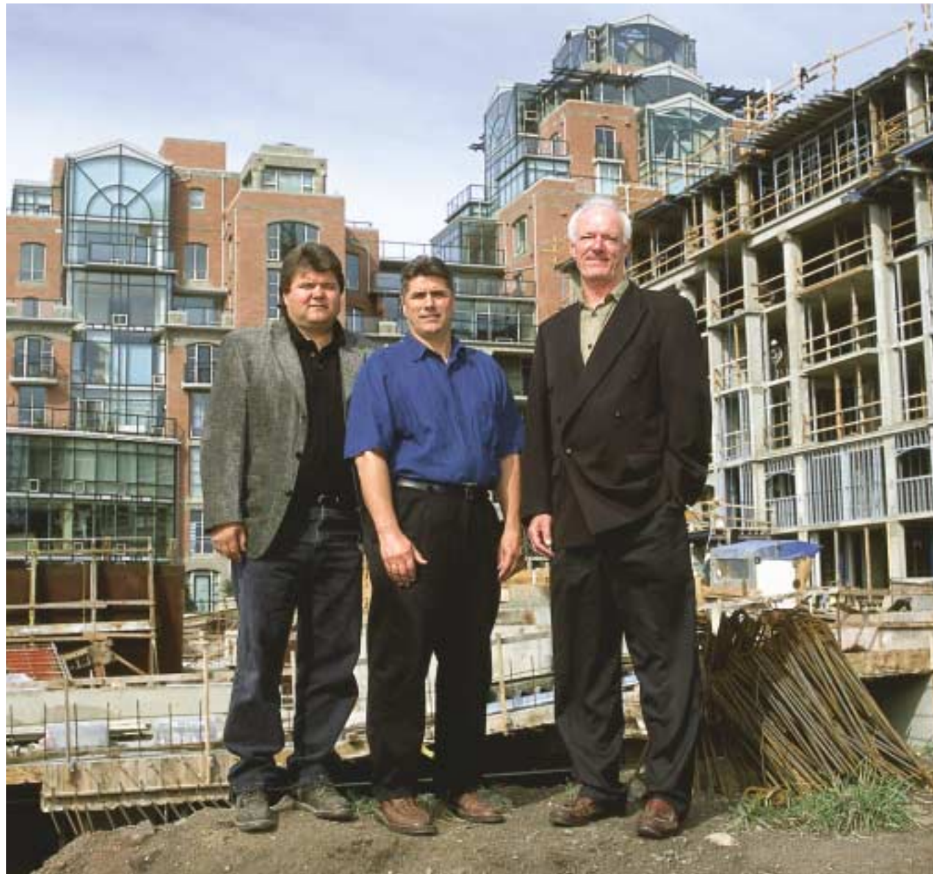
Farmer Construction's 3rd generation owners standing in front of Victoria's luxury Shoal Point Condominium project: (left to right) Lyle Scroggs, Vice President and General Superintendent; Barry Scroggs, Vice President and Contract Estimator and Bill Johnson, P.Eng., President.
