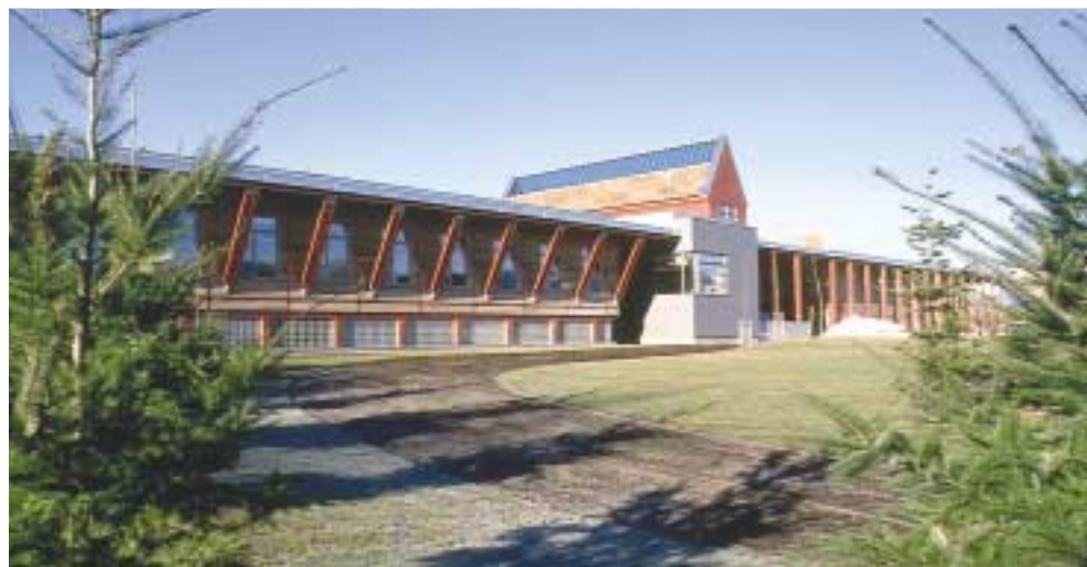
The Forintek Western Research Facility at the University of British Columbia Campus is a showcase of large scale wood product construction. It exemplifies Farmer Construction's commitment to quality and construction innovation.
